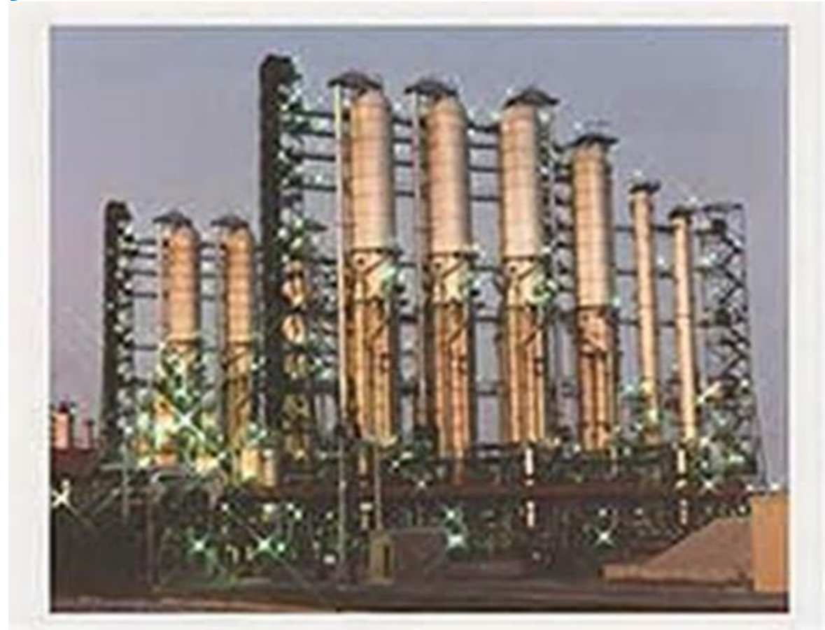
Bruce Heavy Water Plant
