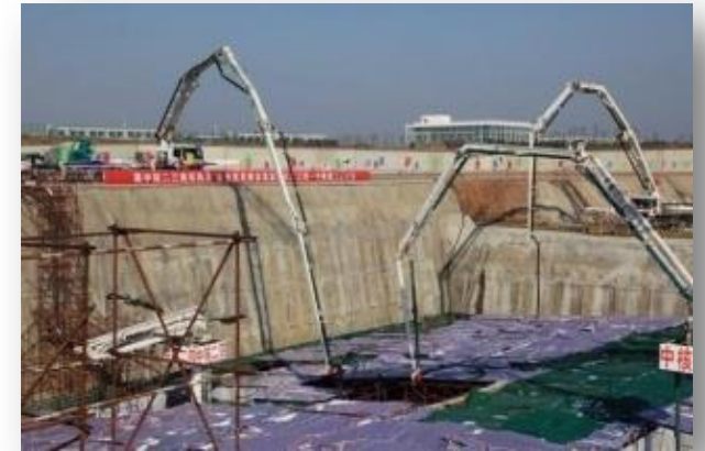
First Concrete poured for China's HTR-PM
