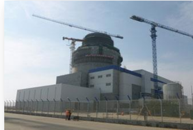
Haiyang – May 2014 Source: State Nuclear Power Engineering
