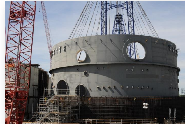
Vogtle – July 2014 Source: Georgia Power Co.
