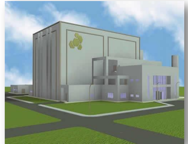
How a power plant based on the CAREM reactor could look (courtesy of Invap)
