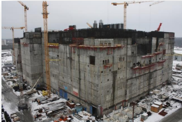
Reactor Compartment of Main Building
