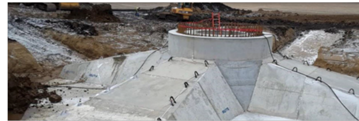
Precast concrete wind turbine foundation (Sargent & Lundy)
