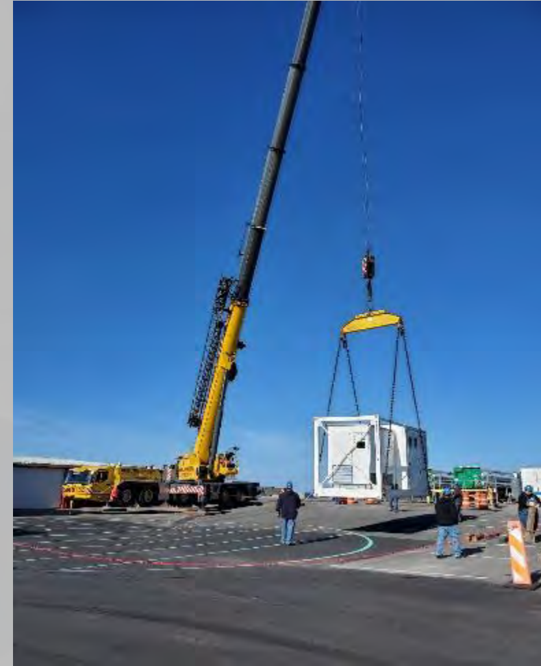
Rigging power supply into place
