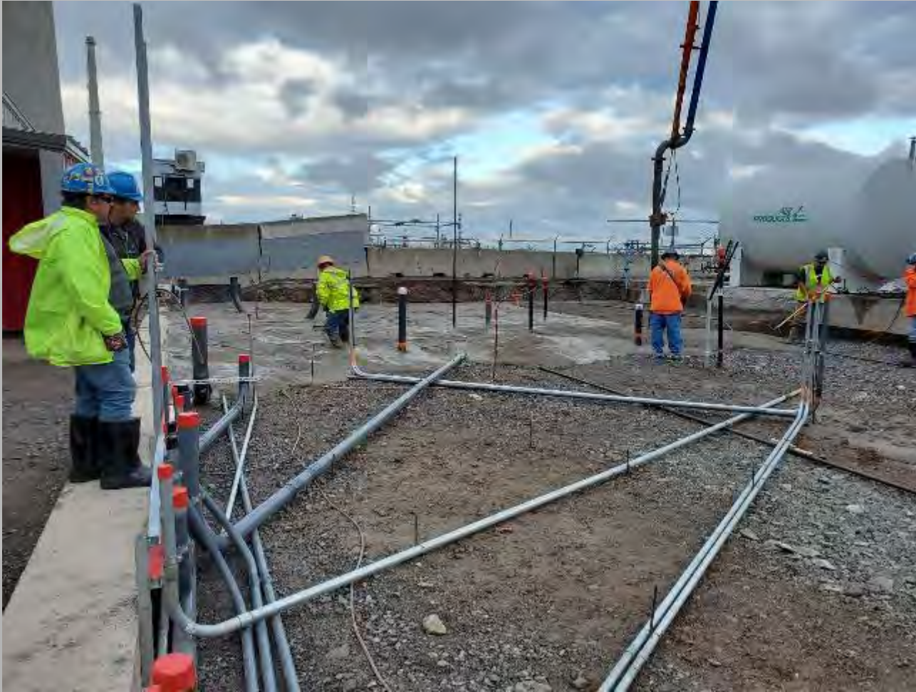
Pouring concrete for electrolyzer
