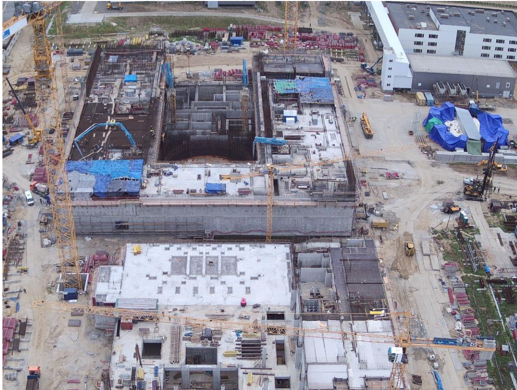
Site (August 2023) View of the reactor building and turbine hall
