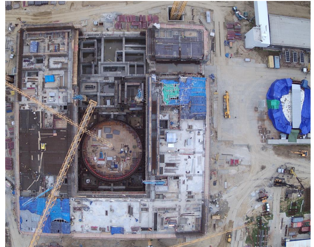
Site (August 2023) Reactor building
